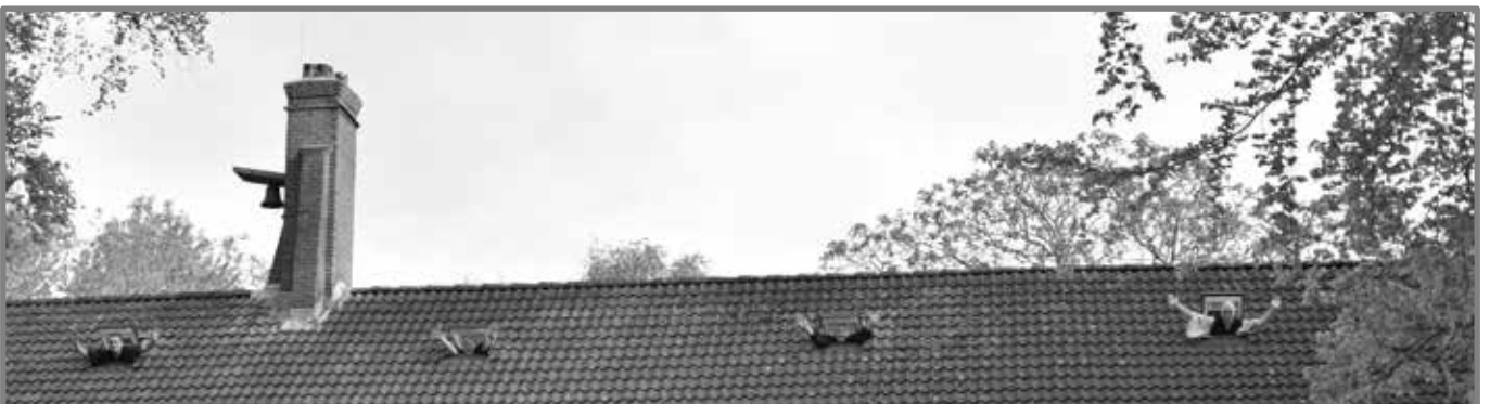
With thanks to Pascal Tetsuko van der Knokke for his help in installing four skylights on the north wing.
